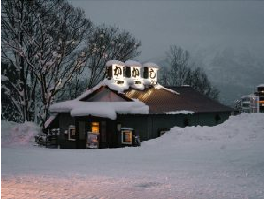
Figure 1: Building Covered with Snow
