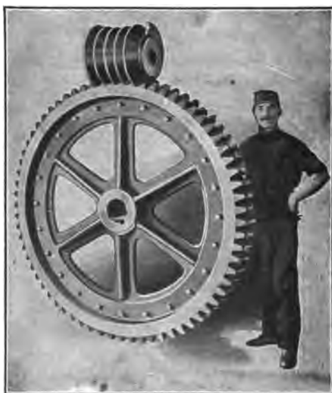
FIG. 108.—This large worm-wheel is a part of the hoisting mechanism employed for the lock gates of the Sault Ste. Marie Canal.
