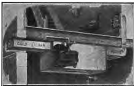
FIG. 144.—Heating by an indirect radiator with side-wall register.
