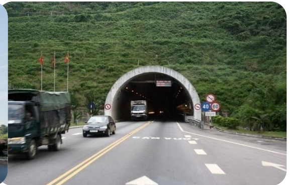
Hai Van tunnel
