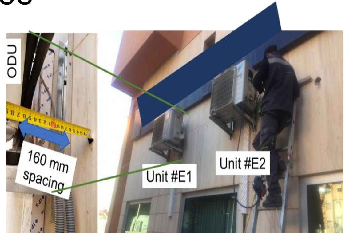
(b) ODUs with good spacing
